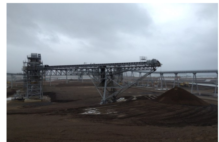
Part of Rikuzentakata's conveyor belt system for moving earth from a neighboring mountain
