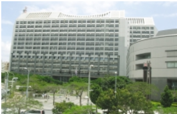
Okinawa government building (left) and the Okinawa Assembly building (right)
